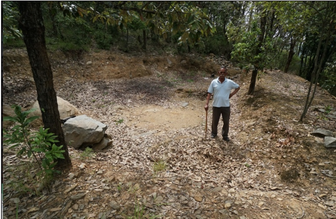
Figure 13. Sarpanch, (main head of forest council), Sir Jagdamba Prasad Joshi stands in the recharge pond. A recharge pond serves as a water harvesting system collecting runoff water from a nearby pine forest and serves as a point of infiltration and groundwater recharge for the Vaishnavi spring. Given a total estimated water storage capacity of 200 m 3 , the pond has the potential to give 0.38 Litres/ha/minute for 365 days. (Photo: HP Liniger)
