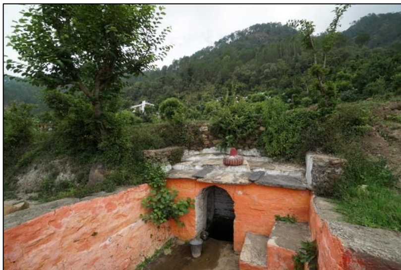
Figure 11. Vaishnavi Naula lies below Nakina's settlement, surrounded by cropland next to the village temple. The Naula is reported to be 1,500 years old and has remained a key source of drinking water. Spring discharge has reduced in the dry season over the last 30 years, but increased in the last two years because of improved forest management and springshed protection. (Photo: HP Liniger)
