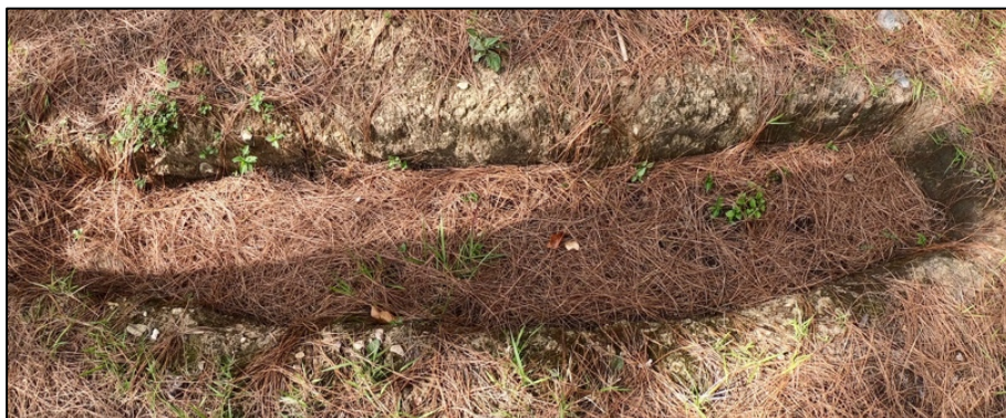
Figure 14. Infiltration trenches established in the recharge zones of a springshed have the potential produce about 0.01 litres per minute per hectare, assuming 957 mm rainfall (30 trenches, 1 meter distance apart, dimensions: 2.5m x 0.25 m x 0.35 m). Cost of labor and maintenance is intensive, as many structures are required to make any substantial contribution to the groundwater recharge. (Photo J Bandy)
