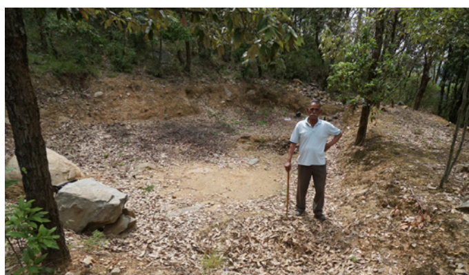
Figure 6. A recharge pond serves as a water harvesting technology, collecting runoff water from a nearby pine forest. It serves as a point of infiltration and groundwater recharge for their local spring. (Photo: HP Liniger)
