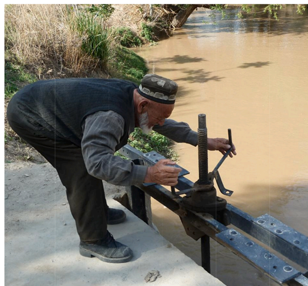
Fig. 7. Rehabilitation of water gates to improve distribution of irrigation water. The breakdown of obsolete water infrastructure caused immense water losses along the canals and the distribution systems in Tajikistan, Aral Sea basin (WOCAT entry n. 1444; https://qcat.wocat.net/en/wocat/technologies/view/technologies_1444/ ).
