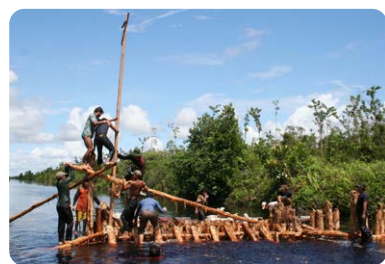
Peatland restoration – blocking drainage channels
