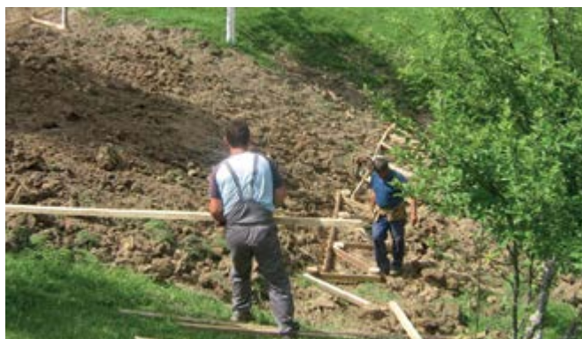
Construction of wooden structures to stop the landslide in Borak, Kladanj municipality. https://qcat.wocat.net/en/wocat/technologies/view/technologies_4285/ https://qcat.wocat.net/en/summary/5190/?as=html
