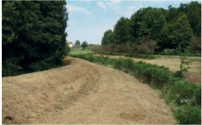
Circumferential (diversion or interception) canals to protect the agricultural area in the plain from mountain waters, Nožičko, Srbac municipality, north Republic of Srpska.
