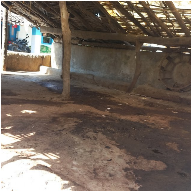
A newly constructed cowshed unit with cement concrete floor (Santosh Gupta)
