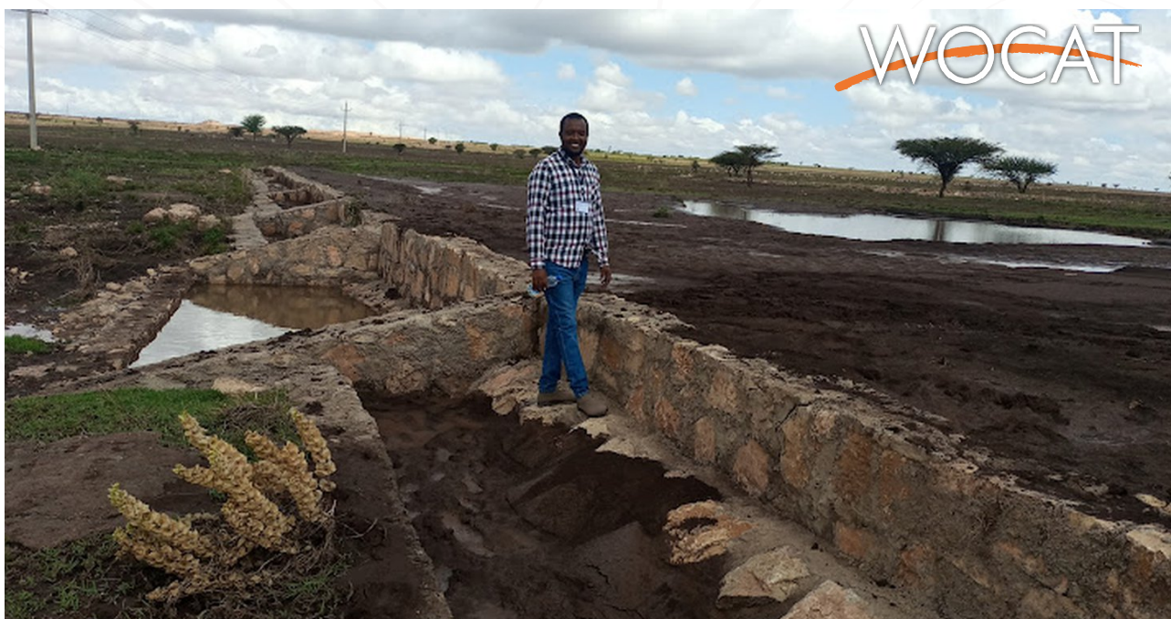
Water Spreading Weirs (WSW) having just arrested fresh sediment and water from upstream runoff in the Togslwro cascade of Amadle kebele, South Jijiga district. (Gerba Leta)
