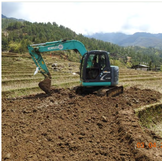
Terrace Consolidation in Progress using an excavator (Tashi Wangdi)
