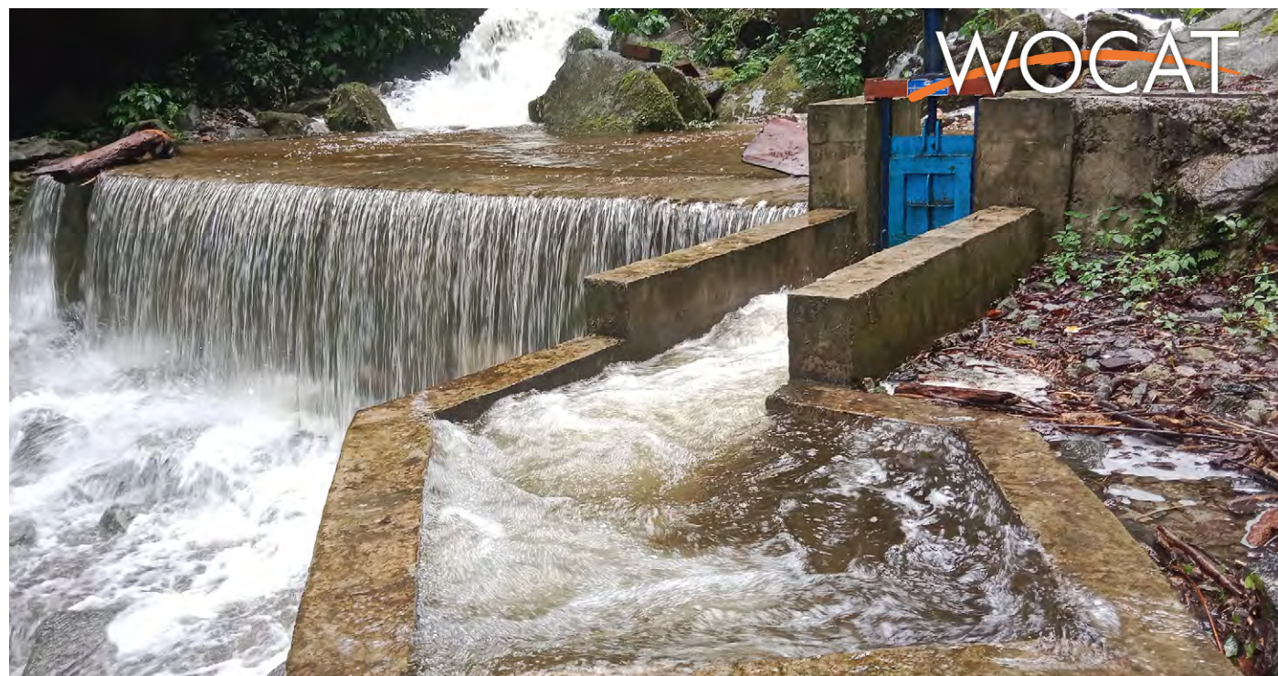
Climate Resilient Irrigation Scheme (sluice gate of the irrigation system) (Kuenzang Nima)
