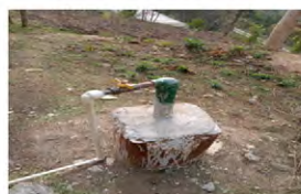
Valve to control amount of gas going to stove
