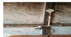
Pressure valve to check pressure of incoming gas from digester
