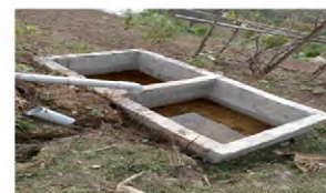
Slurry pit slurry that comes out of digester
