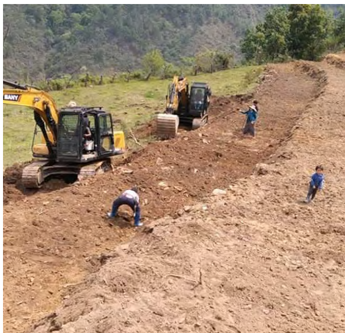
Mechanical bench terracing in progress at Bemji village, Nubigewog (block). (Chenga Tshering)
