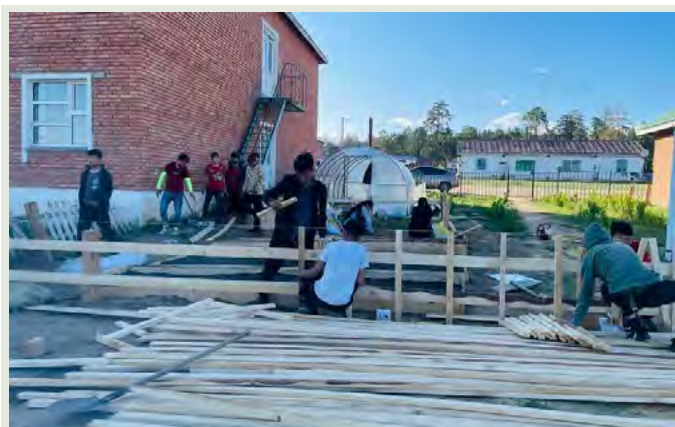
Setting up the fence to surround the soil for planting in the open field. (B. Byambadelger)
