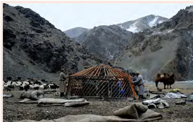
Neighbouring herders working together to erect a ger at a seasonal campsite. They cooperate in assembling the wooden wall frame and roof poles while establishing the new camp. (SEMOON STUDIO)
