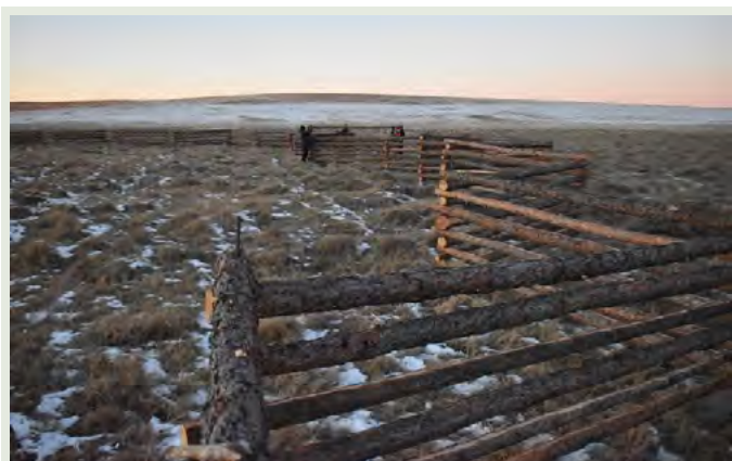
The process of building a Buryat sheep fence (Uuganbayar Munkhbat)
