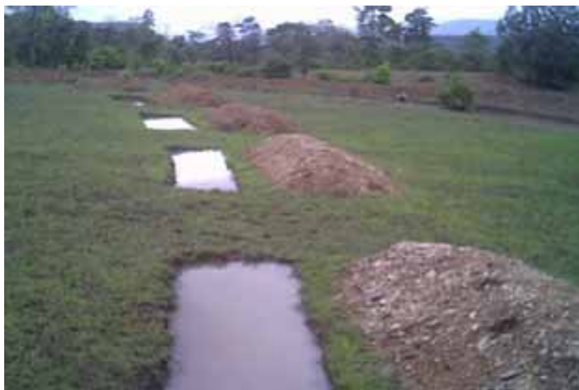
Staggered Contour Trench for Water & Soil Conservation
