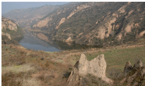
A check dam in the Loess Plateau of China provides and traps sediment until it is filled up. It is then used for crop production. Photo: Hanspeter Liniger
