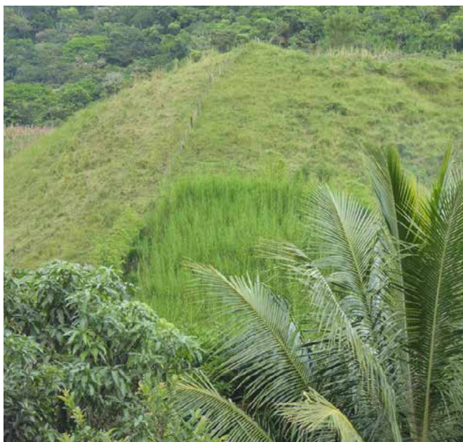
Fascine drains covered with Maralfalfa grasses - a fodder that can be cut and fed to livestock (Helen Gambon, Swiss Red Cross).
