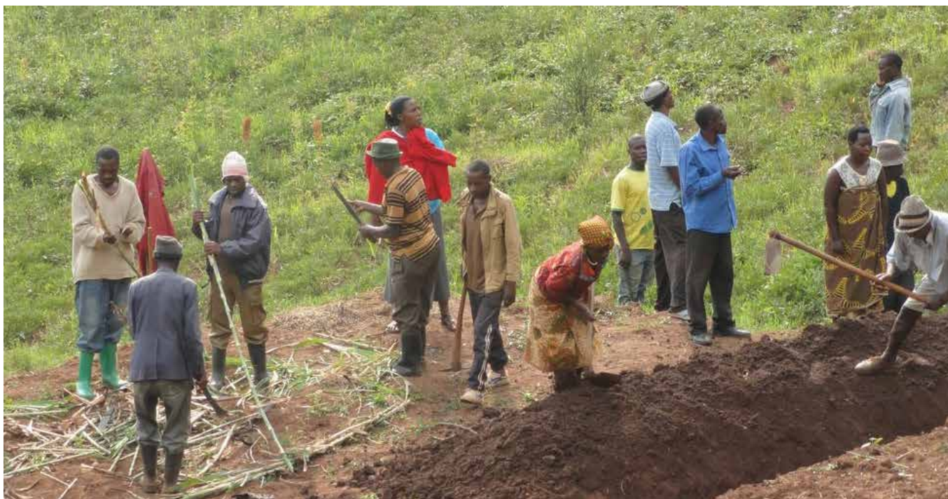
Excavation of soil and water conservation channels with earth ties (Kenneth Twinamasiko).
