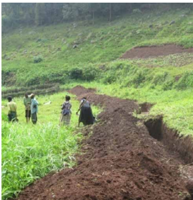
Excavation of soil and water conservation channels separated by earth ties (Kenneth Twinamasiko).
