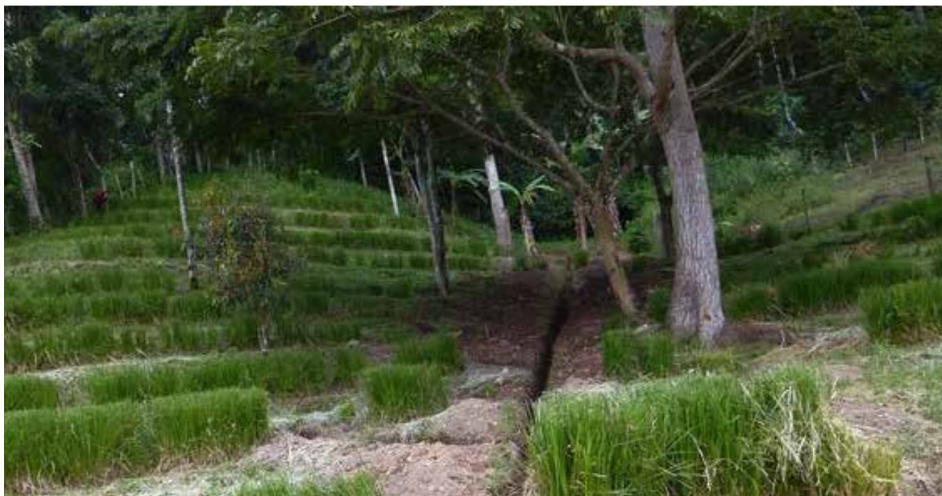
Fishbone shaped ditches ready to be filled with fascine bundles before being covered with soil (Helen Gambon, Swiss Red Cross).
