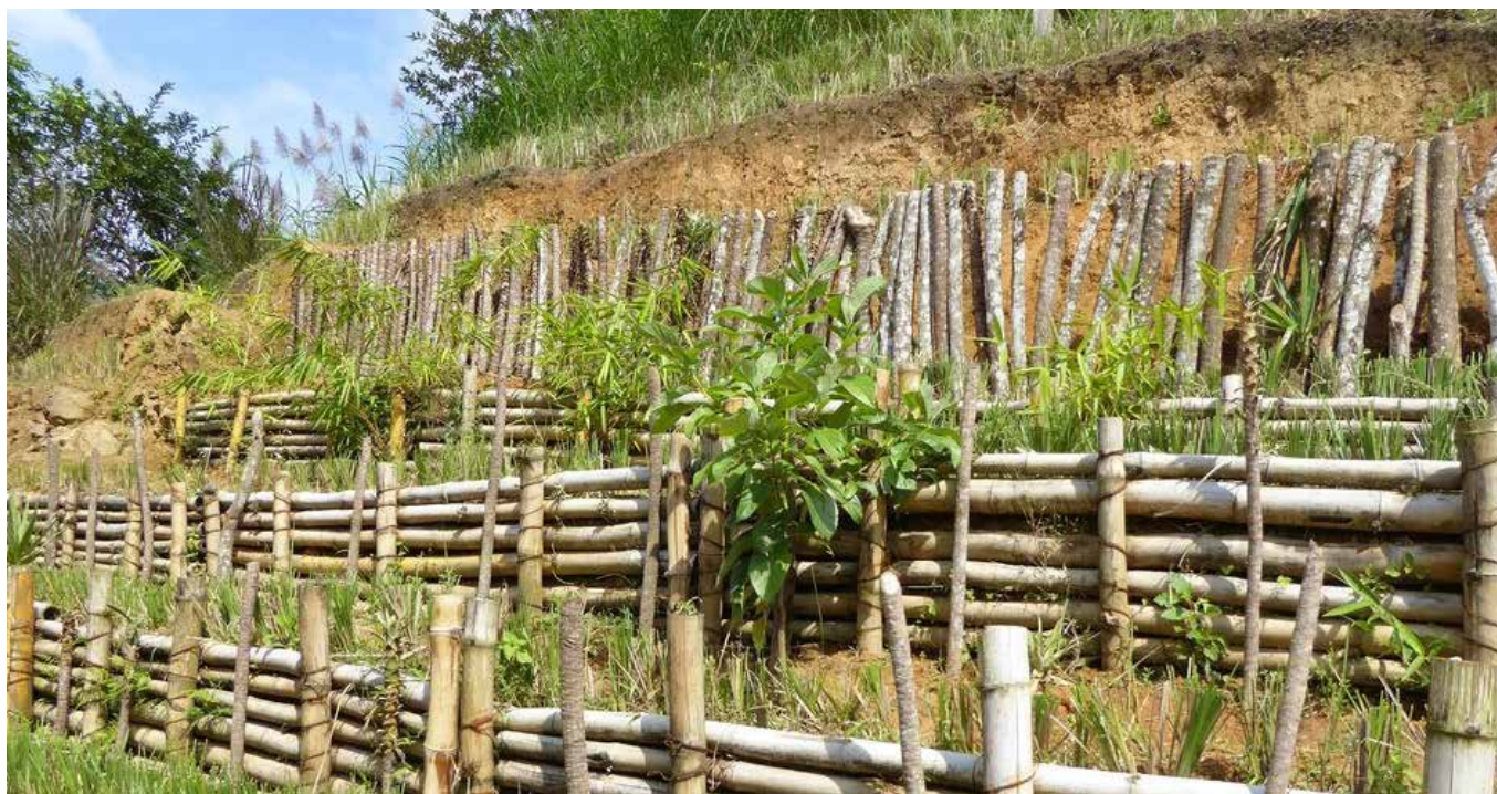
Diverse bioengineering measures are combined to stabilise a slope that poses a risk to a house nearby (Helen Gambon, Swiss Red Cross).
