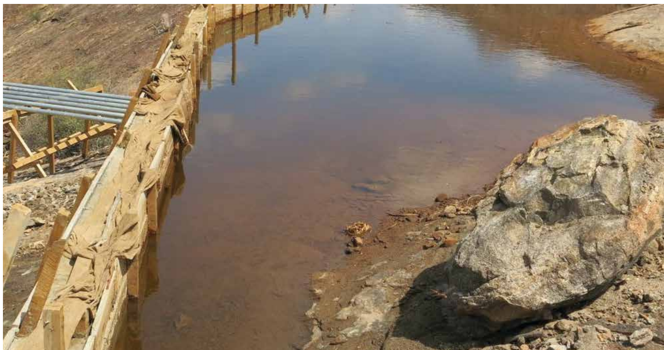
Community rock catchment under construction in Ndirir village, Marsabit County, Kenya. The weir dams hold surface runoff when it rains, channeling the water into a piping system which leads the water into masonry storage tanks (Fredrick Ochieng).
