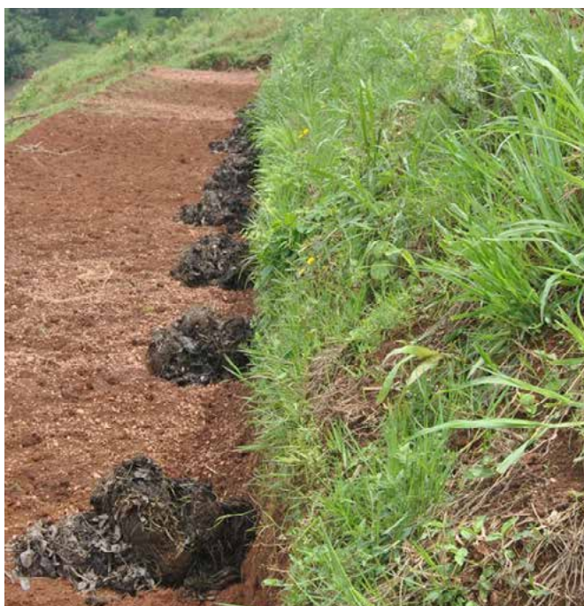
Newly constructed bench terrace planted with grass on the face and lip of the riser for stabilisation (Kenneth Twinamasiko).
