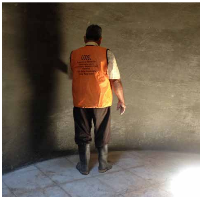
A member of the Local Emergency Committee (CODEL, acronym in Spanish) inside a tank with new flooring and coating (Swiss/Honduran Red Cross).
