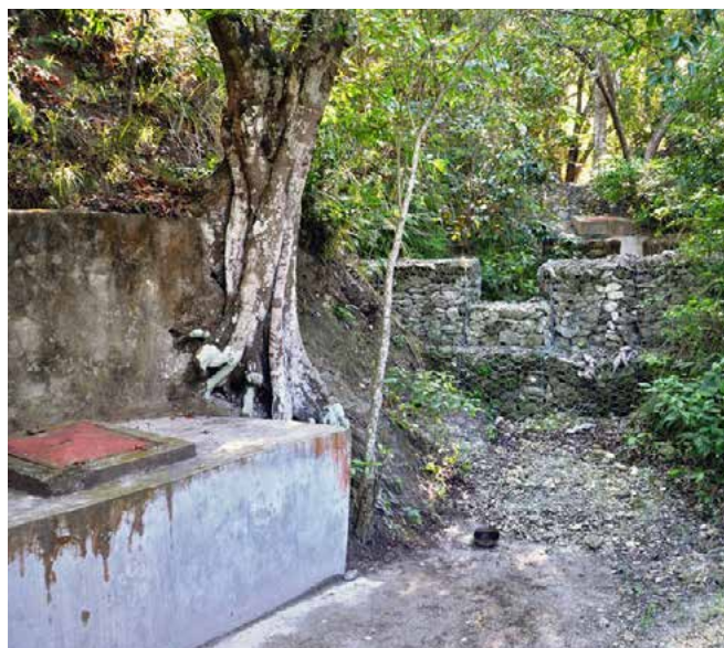
Physical protection of an intake point (in zone 1) (HELVETAS Swiss Intercooperation).
