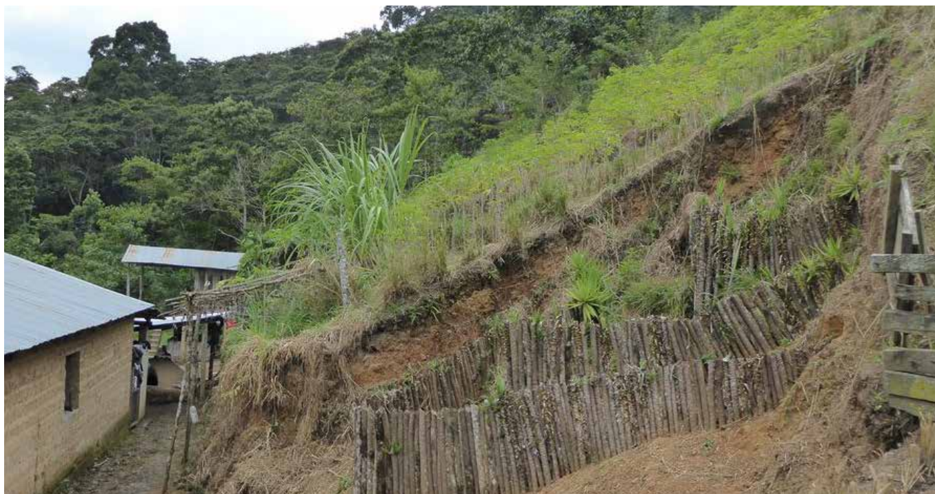
A series of V-shaped catchment fences using izote ( Yucca sp. ) to prevent gully erosion and protect a nearby house. (Helen Gambon, Swiss Red Cross)
