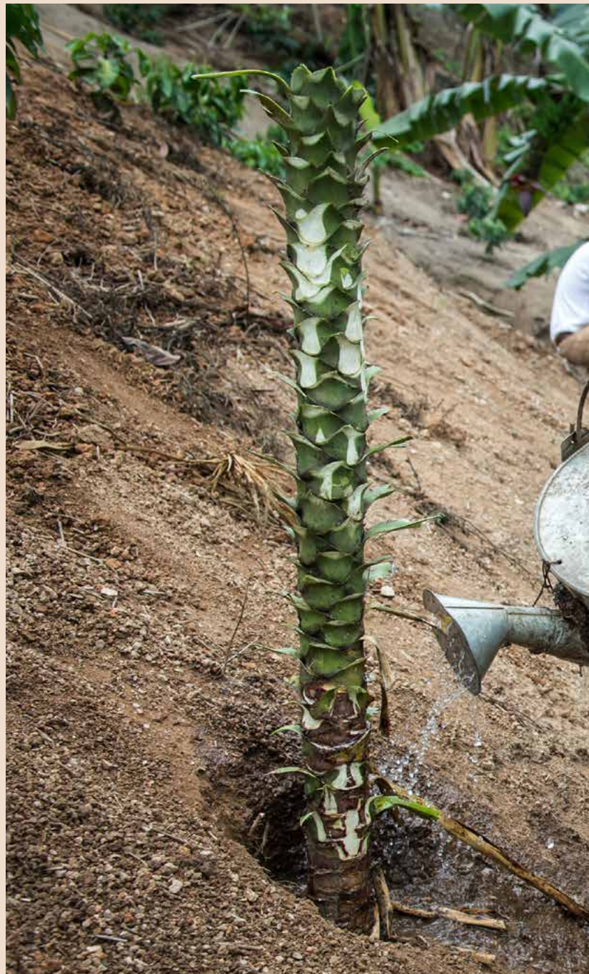
Swiss Red Cross, Honduras – Steep and deforested slopes pose a threat to homesteads; the slopes are stabilised with soil bio-engineering measures such as contour-planting for progressive terracing.
