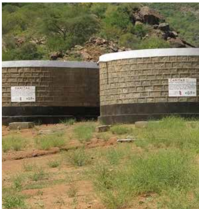
Four masonry tanks each 50 cubic metres in Ndikir Rock catchment (Joy Kivata).
