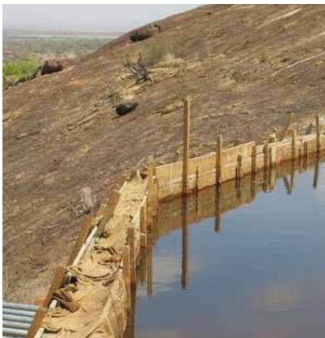
Front part of a weir showing pipelines (Joy Kivata).
