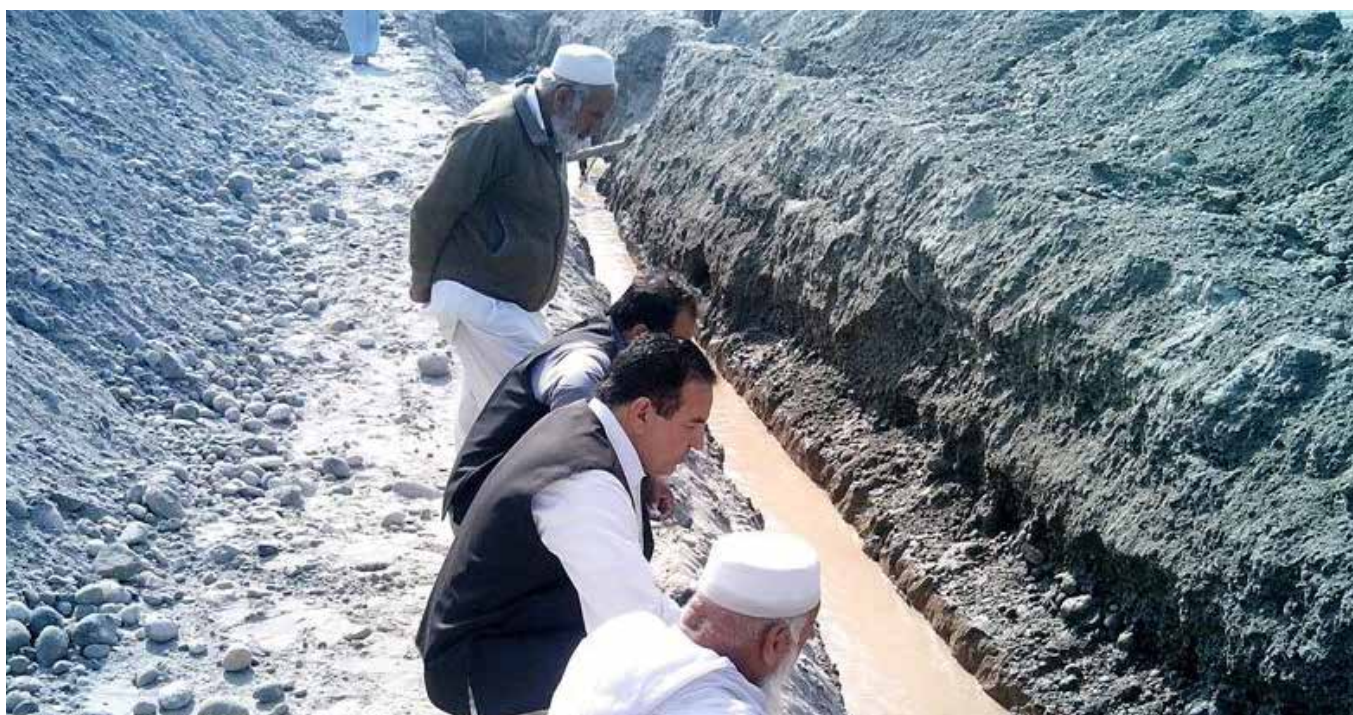
Local actors during a joint inspection of a water-gallery under construction (HELVETAS Swiss Intercooperation Pakistan).
