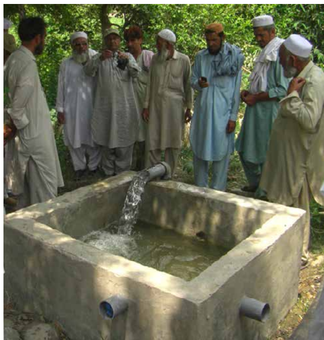
Collection chamber: infiltration gallery system (HELVETAS Swiss Intercooperation Pakistan).
