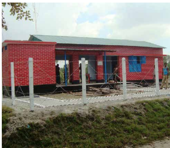
Safety and health at the Community Resource Centre and Community Clinic. The structures are built on an elevated foundation to protect them from floods (Tuhin Samaddar).
