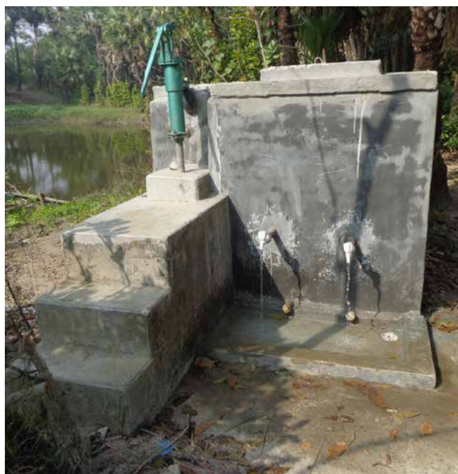
Pond Sand Filter after construction (Md. Saiful, WASH Infrastructure Officer).
