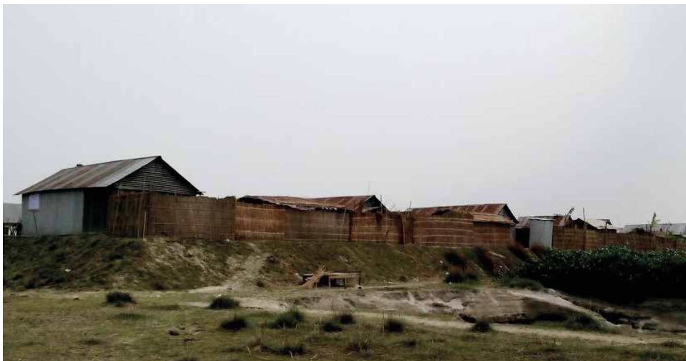
Raised foundations protect emergency infrastructure from floods, providing shelter and access to health and water and sanitation facilities (Tuhin Samaddar).
