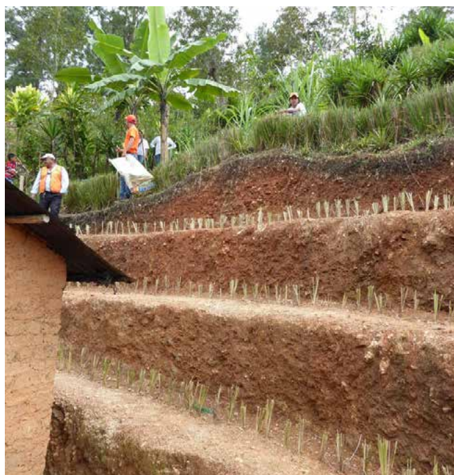
Living barriers of vetiver grass combined with terracing (Helen Gambon, Swiss Red Cross).
