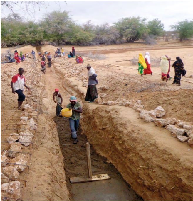
Excavation process (from IUCN archive).
