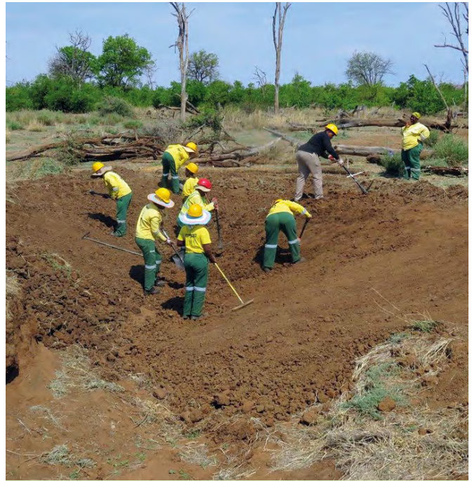
Reshaping of the gully (J Buckle).
