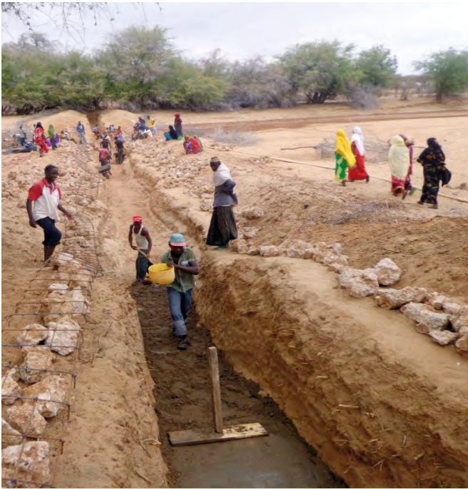
Excavation process (from IUCN archive).
