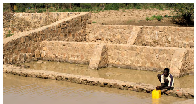
Water-spreading weir, Mali (Klaus Wohlmann).
